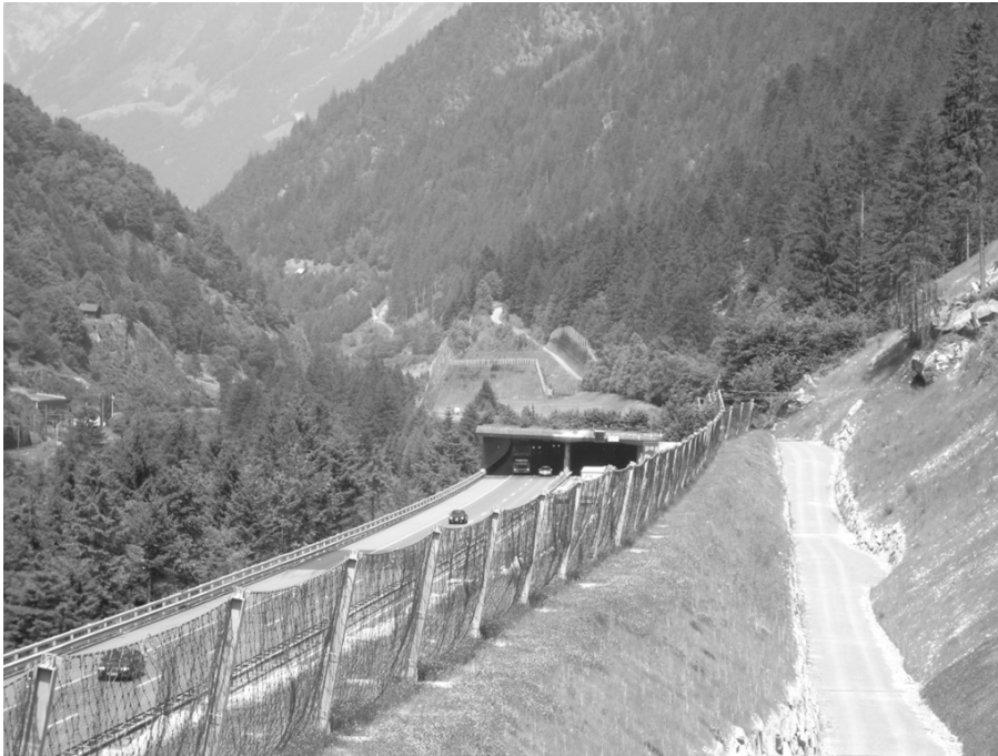
Figure 5.16. Photo showing an 8 m high rock catching dam, with a wire rope net on top protecting against ballistic rock fragments along the Gotthard highway in Switzerland (Photo V. Labiouse)
